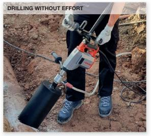
Compact, lightweight drilling system for wet drilling in the sewer. The manual feed is generated by the handwheel and the continuous feed rod.
