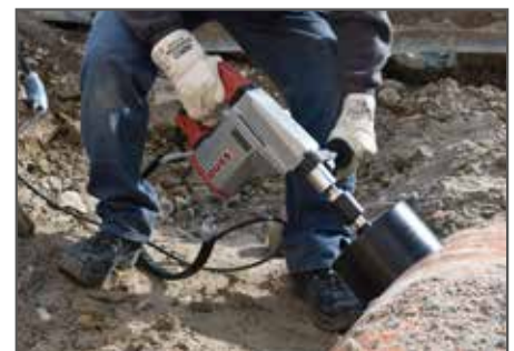
Dry drilling in a plastic pipe, hand held
