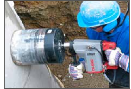
Wet drilling in a concrete shaft, hand-held
