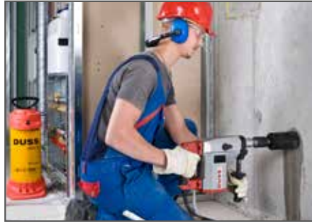
Wet electrical socket sinking in concrete, hand-held
